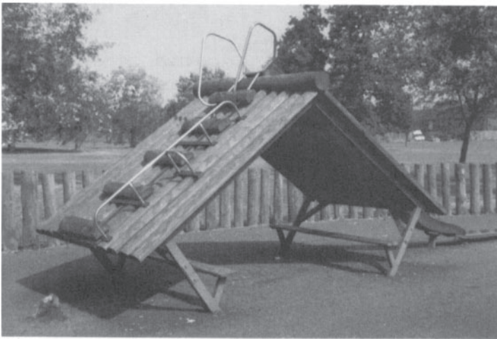
Figure 3.9 Poor maintenance—broken step with sharp point.
